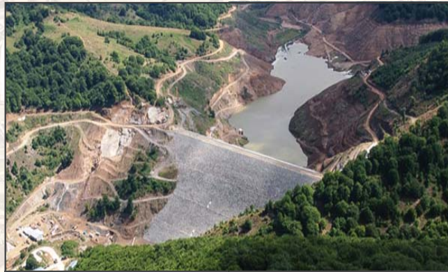
ZLETOVICA DAM - NORTH MACEDONIA
